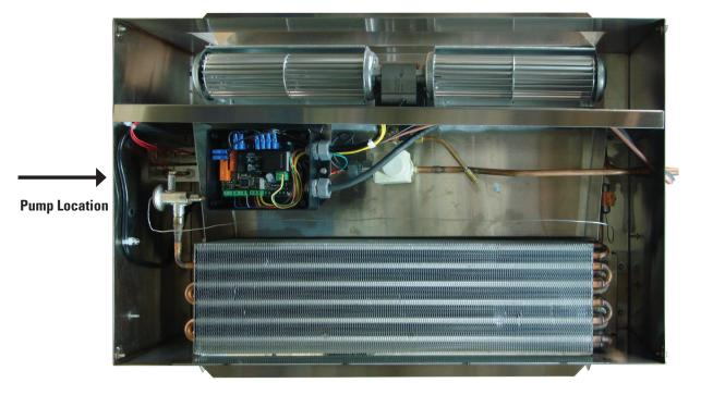
7. Attach the 1/4" vinyl hose drain tube to the outlet of the condensate pump. Run the line to the nearest drain and afix with a clamp. The pump sits flush in the bottom of the sump.
